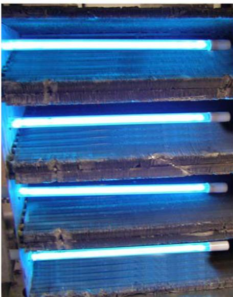
**Example No. 4:** A large residential coil could require nine UV bulbs to provide good UV protection for mold/bacteria growth. This will add approximately 300 watts of heat energy to the air conditioner system. However, the mold/bacteria protection and subsequent air flow savings would make this installation worthwhile.
