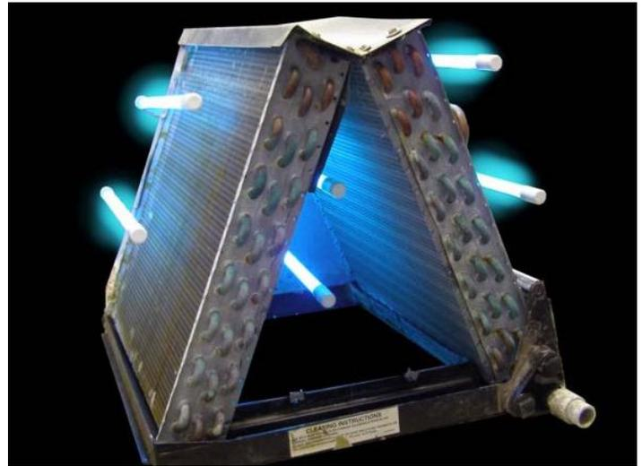
**Example No. 5:** A large residential AC coil will require 6 lamps for a good coverage. This is an example of an excellent installation.
