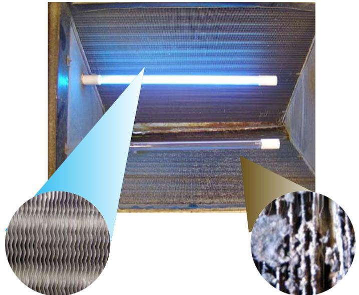
**Example No. 2:** A ten-year old air conditioner coil with a UV bulb placed too close to the end coil. Most of the coil was clean, but the 25% over 8” away grew mold and bacteria actually blocking air flow of 25%. This installation was of some value to the client, but not 100%.
